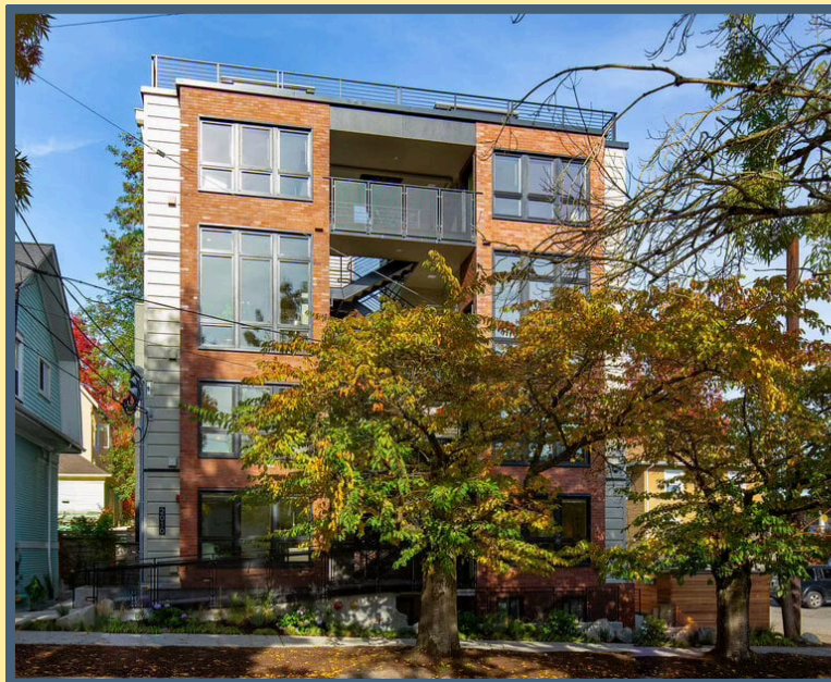
Source: CAST Architecture
